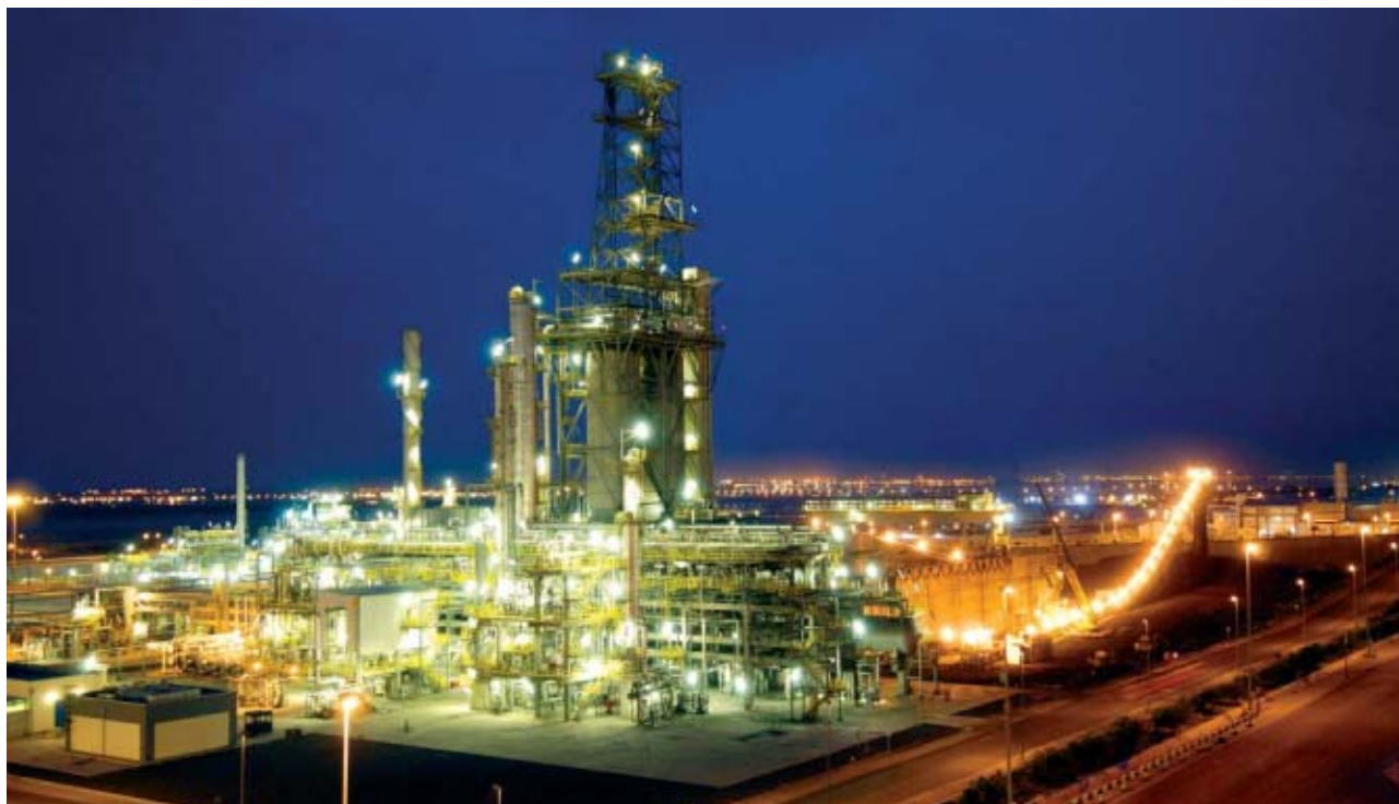
Midor is a grass roots refinery with a design capacity of 100,000 barrels per stream day (b/sd) built around eight licensed units.
