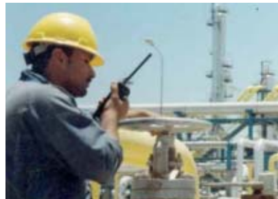
Workers oversee security of plant.
