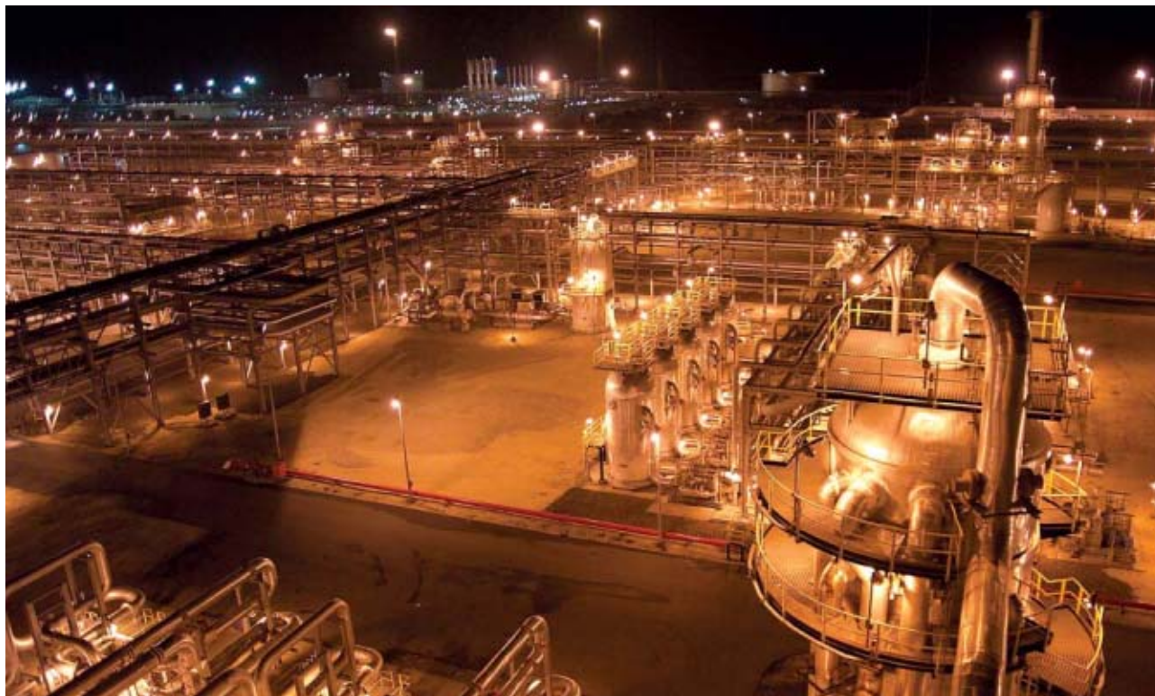
A final element of the natural gas value chain is natural gas liquids. NGLs extracted at a processing plant provide liquefied petroleum gases (LPG).
