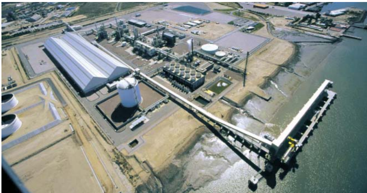
Almost 30 million sq m of land in seven areas has been designated for possible petrochemical projects. Amonia/Urea Complex in Damietta.
