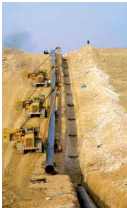
Arab Gas Pipeline, Jordan.
