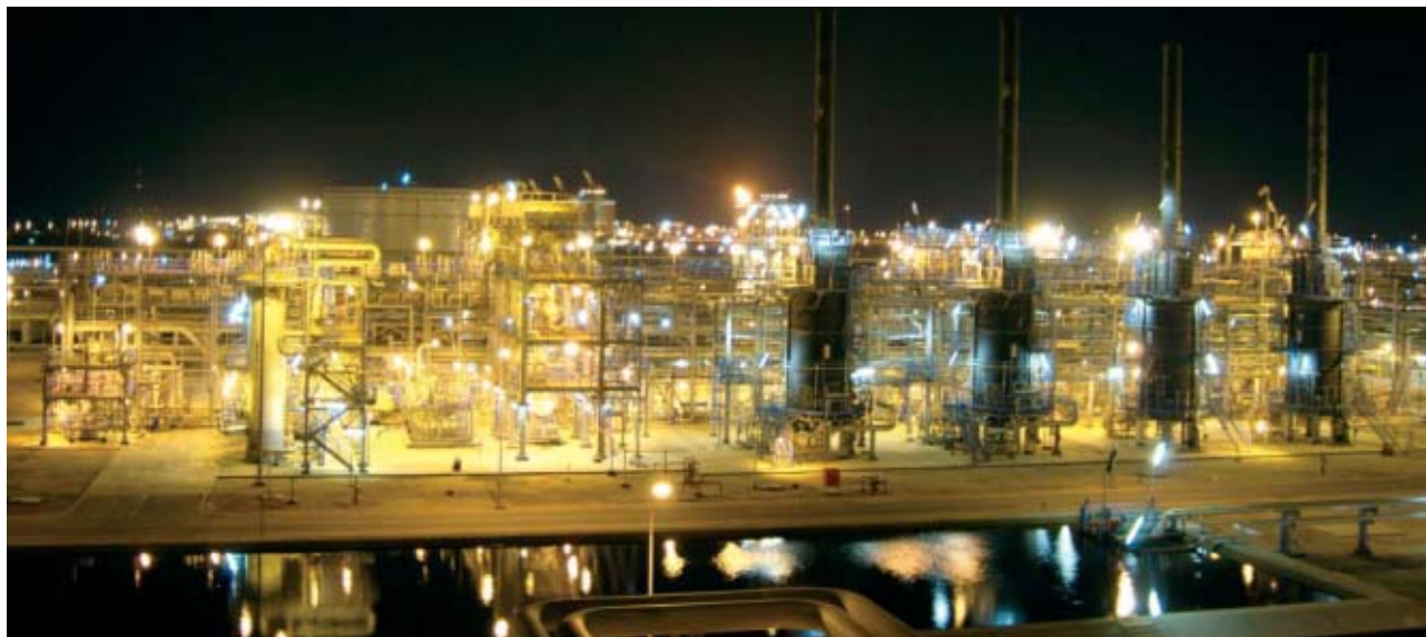
Simian Sienna Gas plant. The bulk of Egyptian gas reserves are in the Nile Delta area and in the Mediterranean.
