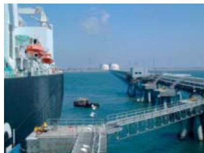
Train 2, Idku Natural Gas Liquefaction Co.
