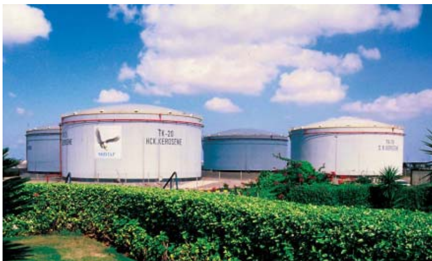
Kerosene storage tanks. Midor refinery produces LPG, 95 (RON) gasoline, jet fuel and diesel.
